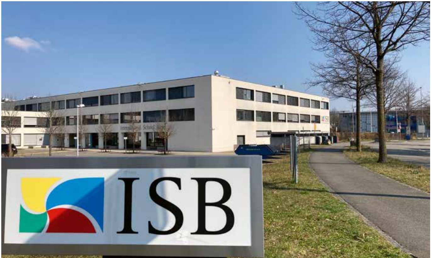
The International School Basel (ISB) disposes of three locations in the canton of Basel-Landschaft (here the ISB in Reinach on Fleischbachstrasse). PHOTO: PATRICK HERR
